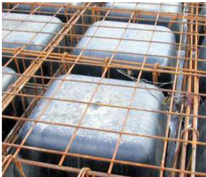
Figure 8. Waffle slab steel placing
